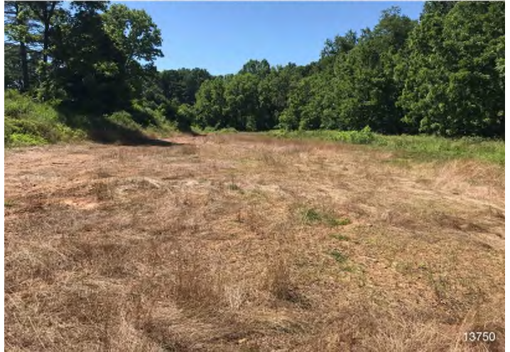
Figure 4: STA 13800+00 – Controls in place and functioning properly. Area stabilized with straw and temp. vegetation.
