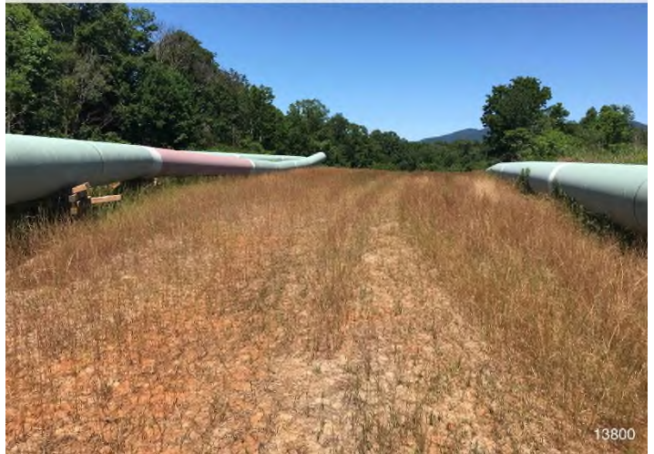
Figure 4: STA 13800+00 – Controls in place and functioning properly. Area stabilized with straw and temp. vegetation.
