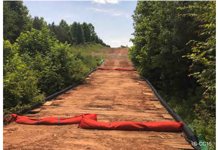
Figure 4: STA 15580+00 – Controls in place and functioning properly. Area stabilized with Earth Guard and straw.
