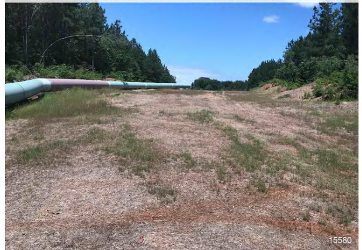
Figure 4: STA 15580+00 – Controls in place and functioning properly. Area stabilized with Earth Guard and straw.
