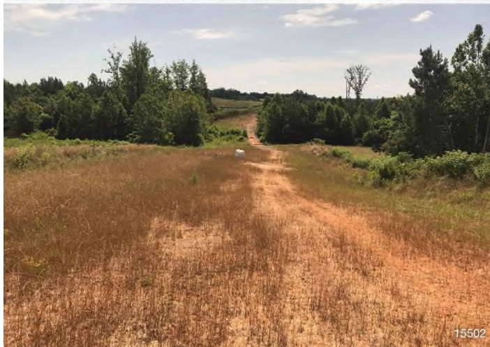
Figure 3: STA 15502+00 – Controls in place and functioning properly. Area stabilized with Earth Guard and straw.
