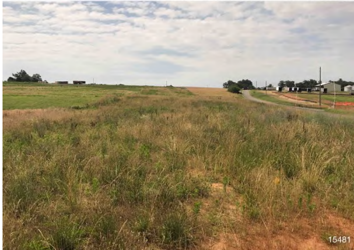
Figure 3: STA 15502+00 – Controls in place and functioning properly. Area stabilized with Earth Guard and straw.
