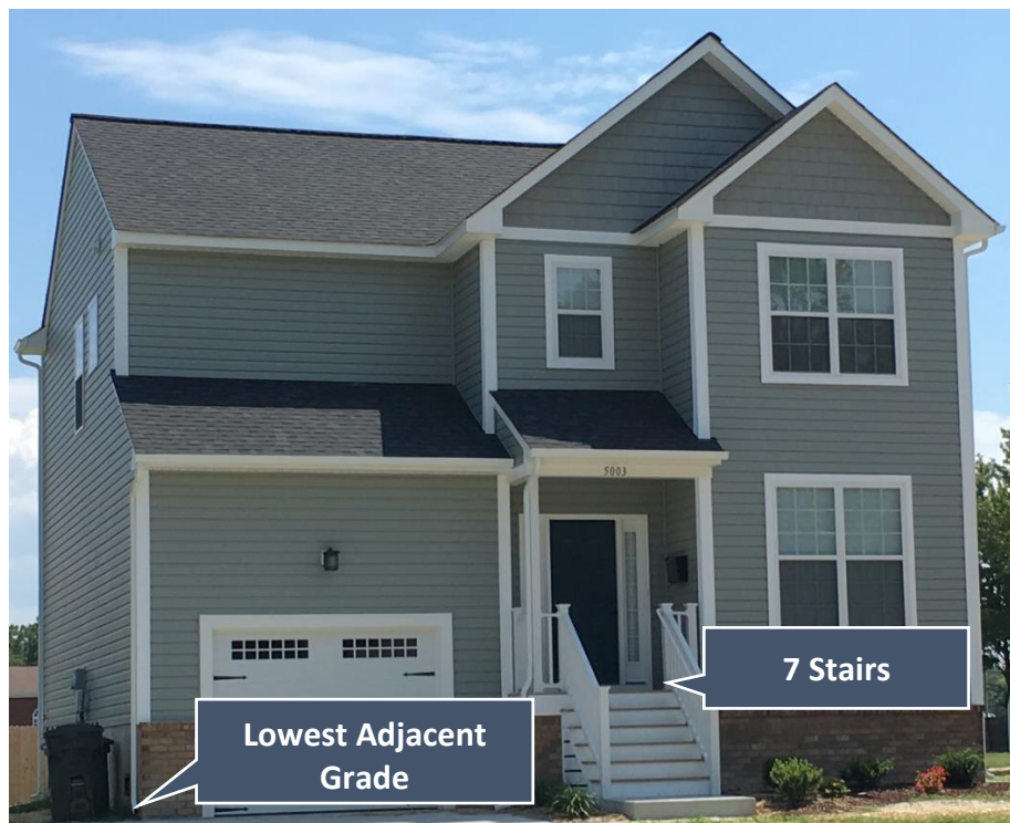
Figure 3: Illustration of stair counting approach for estimating FFH. The count of 7 stairs equals a FFH of 4.4ft. The land elevation difference between the bottom of the stairs and lowest adjacent grade would be added to produce the final FFH estimate. Image from City of Hampton Property Information Parcel Viewer (2017).
