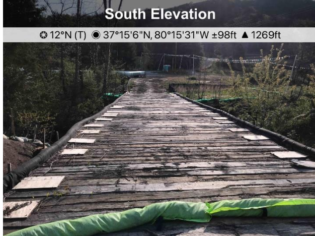
Figure 1: Designated crossing S-C21, ECD's are in place.
