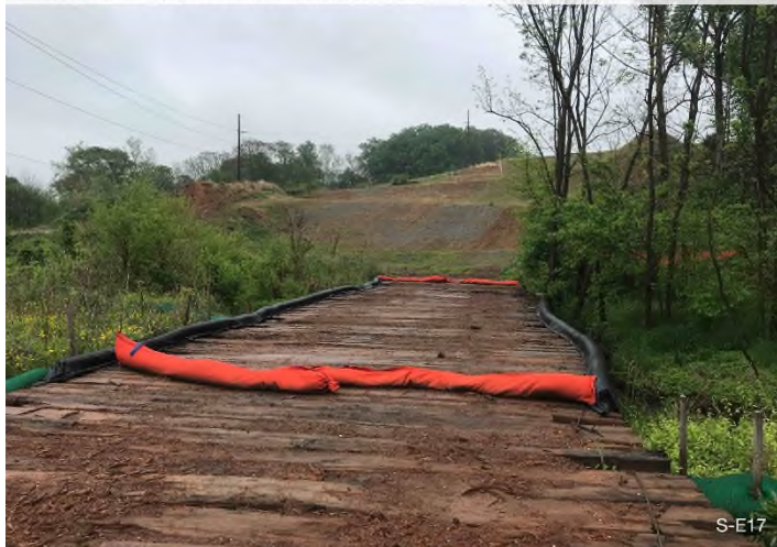
Figure 3: Stream S-E17 – Controls in place and functioning properly around stream crossing.
