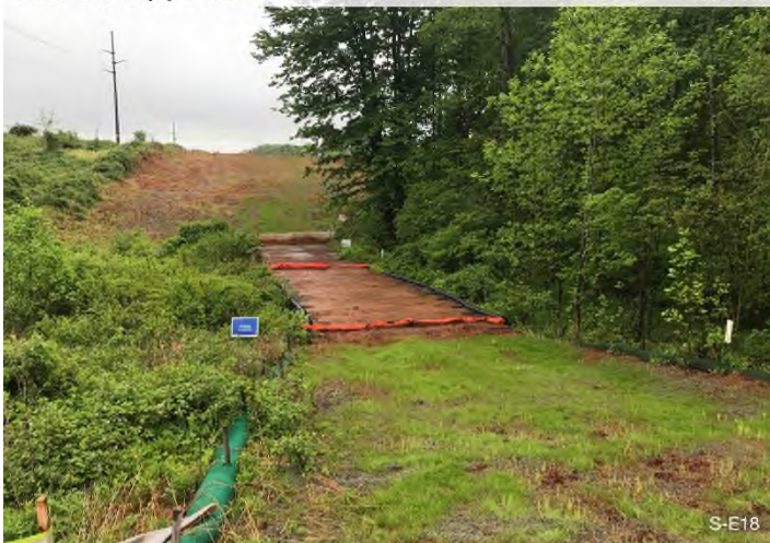
Figure 2: Stream S-E18 – Controls in place and functioning properly around stream crossing.
