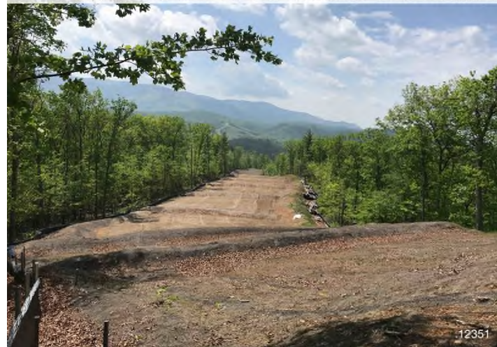
Figure 4: STA 12351+00 – Controls in place and functioning properly. Area stabilized with erosion matting.
