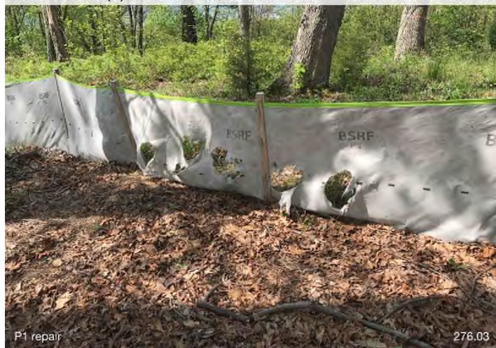
Figure 3: STA 12335+00 – Controls in place and functioning properly. Area stabilized with erosion matting.
