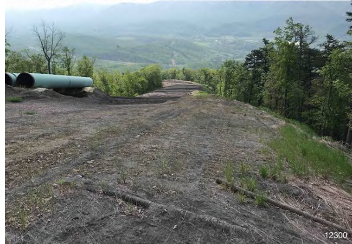
Figure 2: STA 12300+00 – Controls in place and functioning properly. Area stabilized with erosion matting.
