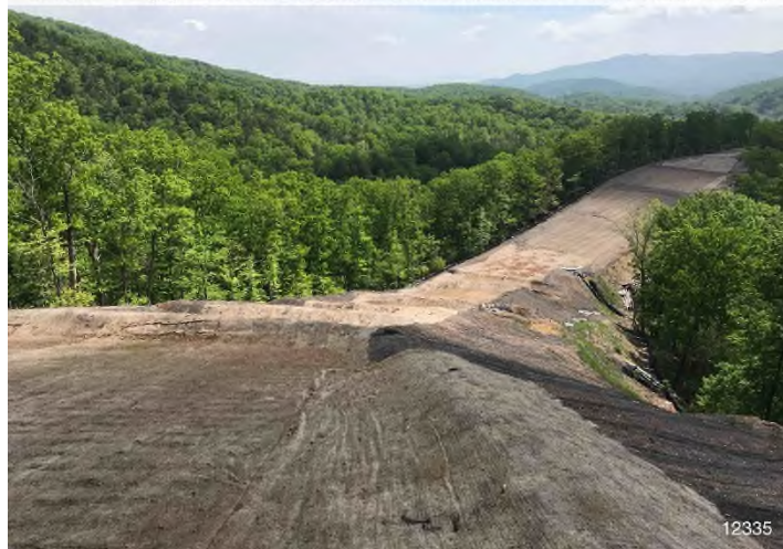
Figure 3: STA 12335+00 – Controls in place and functioning properly. Area stabilized with erosion matting.
