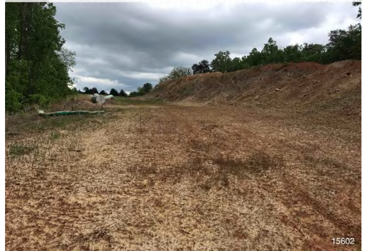
Figure 4: STA 15602+00 – Controls in place and functioning properly. Area stabilized with Earth-Guard. BRG: 91°E (T) LAT: 36.892507 LON: -79.438882 ±13593ft ALT: 813ft
