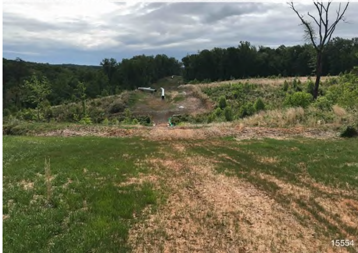
Figure 3: STA 15554+00 – Controls in place and functioning properly. Area stabilized with Earth-Guard. BRG: 118°SE (T) LAT: 36.896103 LON: -79.451283 ±13586ft ALT: 841ft
