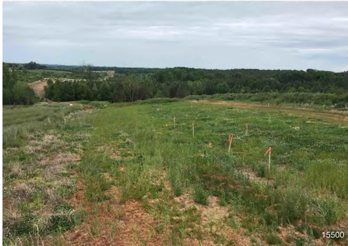
Figure 1: STA 15500+00 – Controls in place and functioning properly. Area stabilized with Earth-Guard. BRG: 149°SE (T) LAT: 36.906191 LON: -79.474077 ±16ft ALT: 927ft
