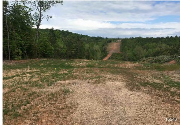
Figure 2: STA 15548+00 – Controls in place and functioning properly. Area stabilized with Earth-Guard. BRG: 304°NW (T) LAT: 36.898366 LON: -79.461016 ±32ft ALT: 796ft
