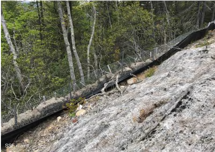
Figure 3: STA 12662+00 – SSF maintenance needed.
