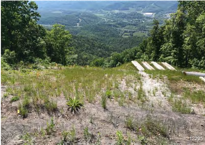
Figure 1: STA 12285+00 – Controls in place and functioning properly. Area stabilized with erosion control matting. BRG: 135°SE (T) LAT: 37.255202 LON: -80.230698 ±164ft ALT: 3149ft
