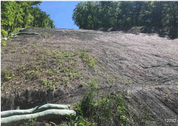
Figure 3: STA 12292+00 – Controls in place and functioning properly. Area stabilized with erosion control matting. BRG: 44°NE (T) LAT: 37.254998 LON: -80.228017 ±32ft ALT: 2281ft
