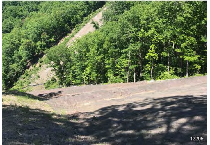
Figure 4: STA 12295+00 – Controls in place and functioning properly. Area stabilized with erosion control matting. BRG: 262°W (T) LAT: 37.255363 LON: -80.226695 ±328ft ALT: 2391ft
