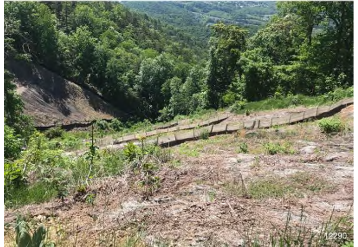
Figure 2: STA 12290+00 – Controls in place and functioning properly. Area stabilized with erosion control matting. BRG: 135°SE (T) LAT: 37.254997 LON: -80.228838 ±32ft ALT: 2407ft
