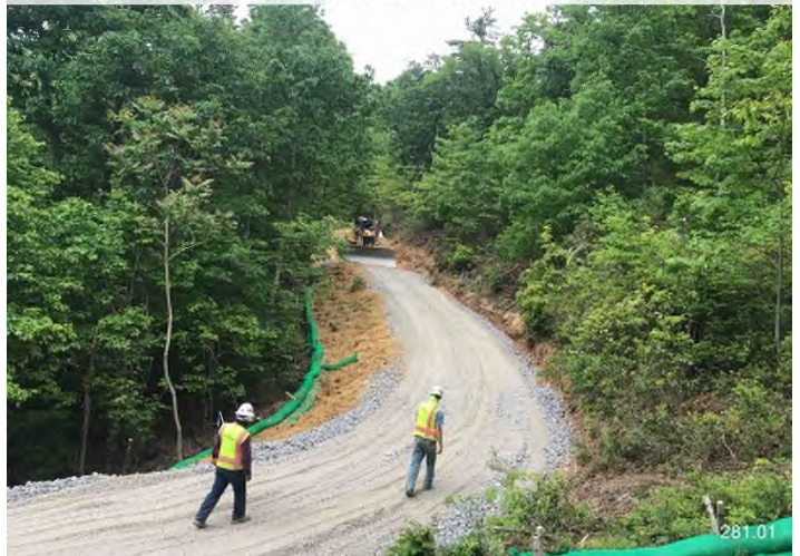
Figure 4: MVP-RO-281 – Controls in place and functioning properly. PPL installing MVP-RO-281.01.
