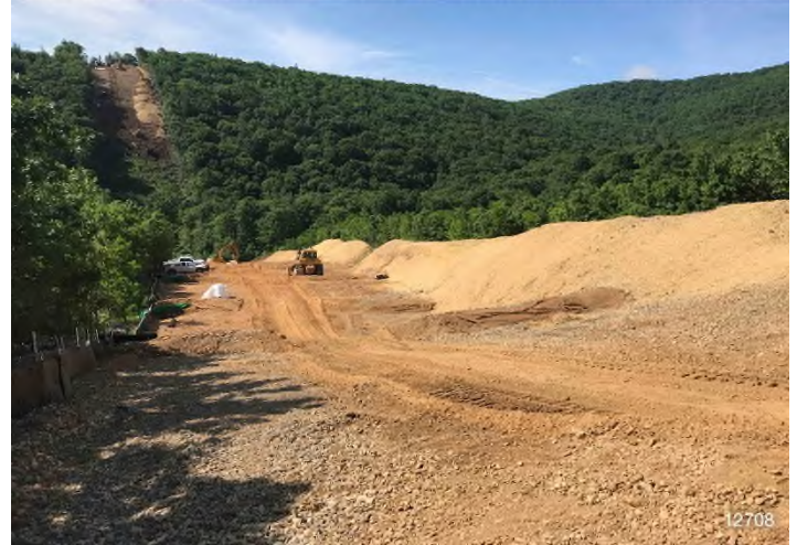
Figure 2: STA 12708+00 – Controls in place and functioning properly. BRG: 182°S (T) LAT: 37.189582 LON: -80.151996 ±98ft ALT: 3069ft
