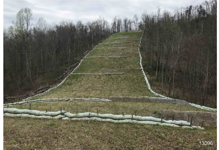
Figure 2: STA 13096+00 – Controls in place and functioning properly.
