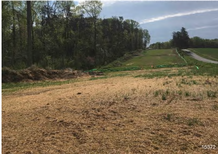
Figure 1: STA 15372+00 – Controls in place and functioning properly. Area stabilized with Earth-Guard and straw. BRG: 118°SE (T) LAT: 36.922348 LON: -79.510340 ±16ft ALT: 780ft
