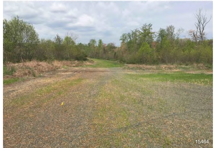
Figure 4: STA 15464+00 – Controls in place and functioning properly. Area stabilized with Earth-Guard and straw. BRG: 295°NW (T) LAT: 36.912470 LON: -79.482609 ±98ft ALT: 1059ft
