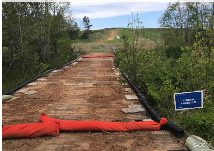
Figure 3: Stream S-CC14 – Controls in place and functioning properly. BRG: 288°W (T) LAT: 36.905344 LON: -79.471385 ±16ft ALT: 872ft
