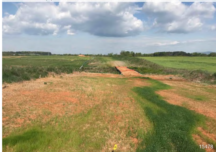
Figure 1: STA 15478+00 – Controls in place and functioning properly. Area stabilized with Earth-Guard and straw. BRG: 226°SW (T) LAT: 36.945758 LON: -79.466987 ±11900ft ALT: 895ft
