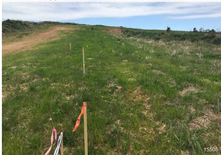
Figure 2: STA 15505+00 – Controls in place and functioning properly. Area stabilized with Earth-Guard and straw. BRG: 298°NW (T) LAT: 36.905558 LON: -79.472466 ±16ft ALT: 880ft
