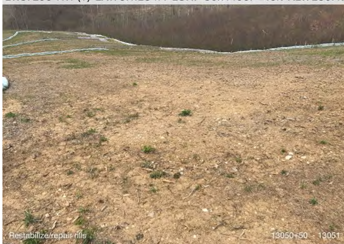
Figure 3: STA 13050+50 to 13051+00 – Re-stabilization needed.
