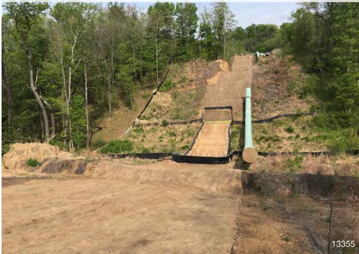
Figure 3: STA 13455+00 – Controls in place and functioning properly. Area stabilized with erosion matting.
