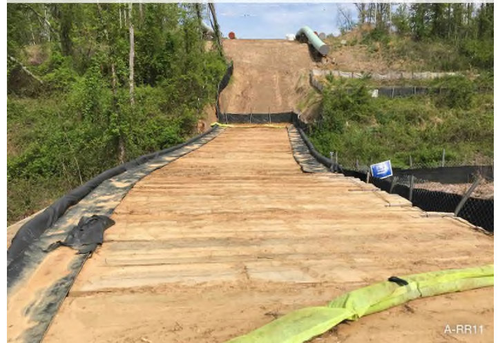
Figure 4: Stream S-RR11 – Controls in place and functioning properly.
