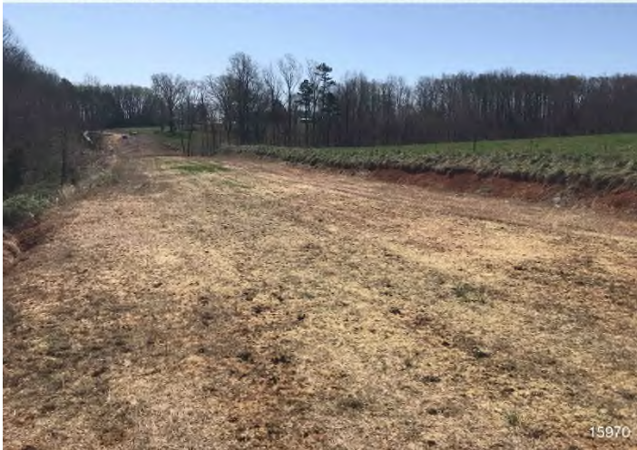
Figure 3: STA 15970+00 – Controls in place and functioning properly. Area stabilized with straw and hydro-mulch. BRG: 156°SE (T) LAT: 36.831479 LON: -79.358222 ±98ft ALT: 622ft
