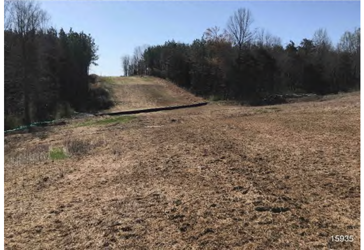
Figure 2: STA 15935+00 – Controls in place and functioning properly. Area stabilized with straw and hydro-mulch. BRG: 167°S (T) LAT: 36.814334 LON: -79.356787 ±24673ft ALT: 638ft
