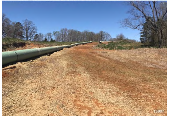
Figure 4: STA 15997+00 – Controls in place and functioning properly. Area stabilized with straw and hydro-mulch. BRG: 263°W (T) LAT: 36.827102 LON: -79.351302 ±16ft ALT: 606ft
