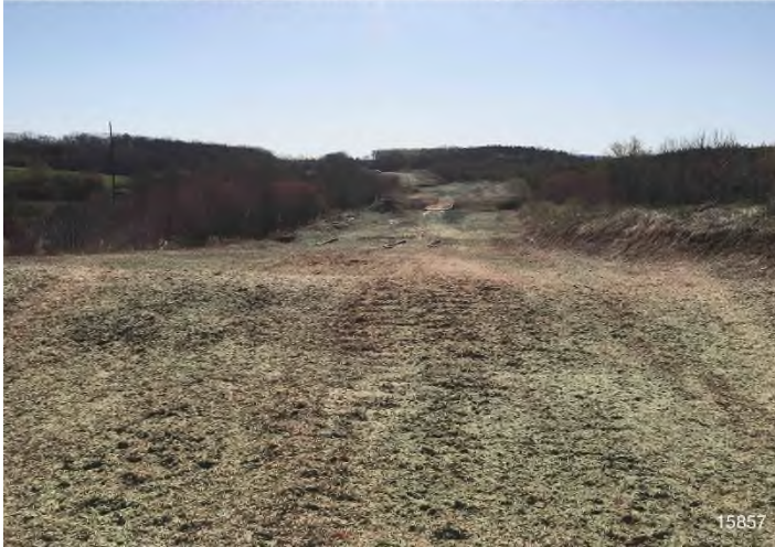
Figure 1: STA 15857+00 – Controls in place and functioning properly. Area stabilized with straw and hydro-mulch. BRG: 116°SE (T) LAT: 36.851358 LON: -79.384242 ±32ft ALT: 739ft
