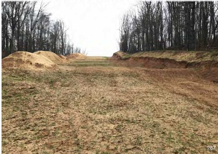
Figure 3: MVP-RO-287 – Controls in place and functioning properly. BRG: 8°N (T) LAT: 37.134932 LON: -80.137876 ±16ft ALT: 2694ft
