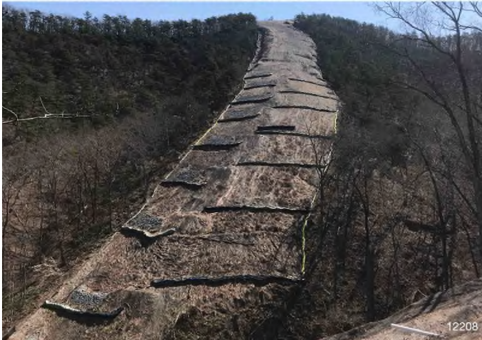
Figure 3: STA 12208+00 – Controls in place and functioning properly.
