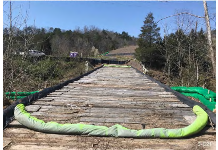
Figure 4: Stream S-C21 – Controls in place and functioning properly around Bradshaw Creek Crossing.
