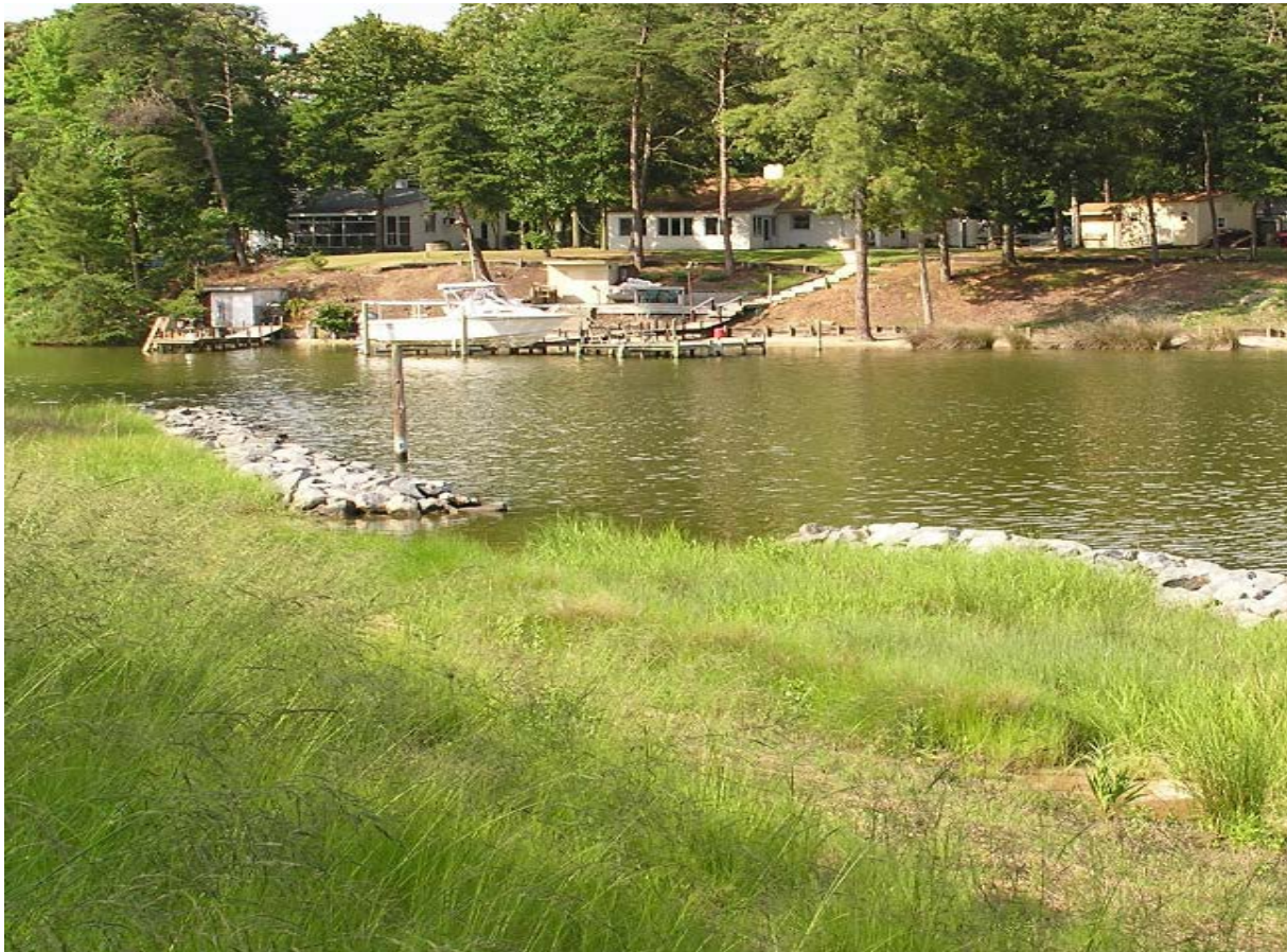
The far shore shows a traditional bulkhead with remnants of a fringe marsh. As the sea level rises, this marsh has nowhere to migrate and will be lost. The near shore shows a living shoreline with a gap in the rock sill to provide water access to the newly created marsh. A graded bank behind this marsh will allow marsh migration. (Photo: VIMS)
