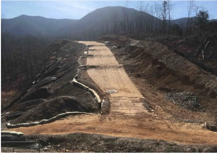
Figure 3: STA 12513+00 – Controls in place and functioning properly. Area stabilized with erosion control matting.
