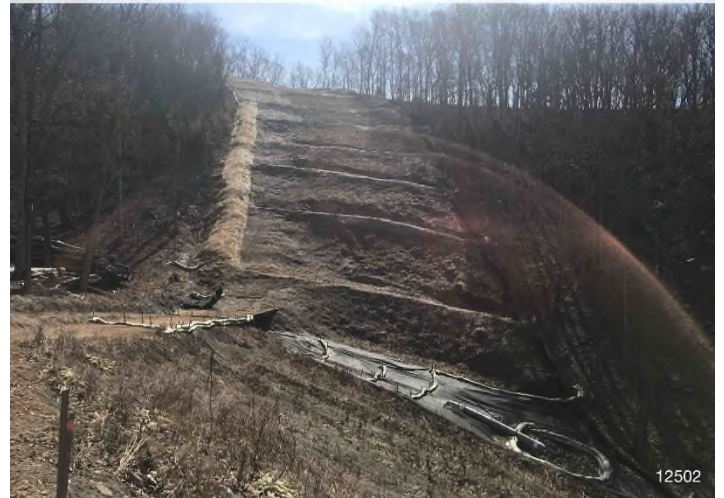
Figure 4: STA 12502+00 – Controls in place and functioning properly. Area stabilized with erosion control matting.
