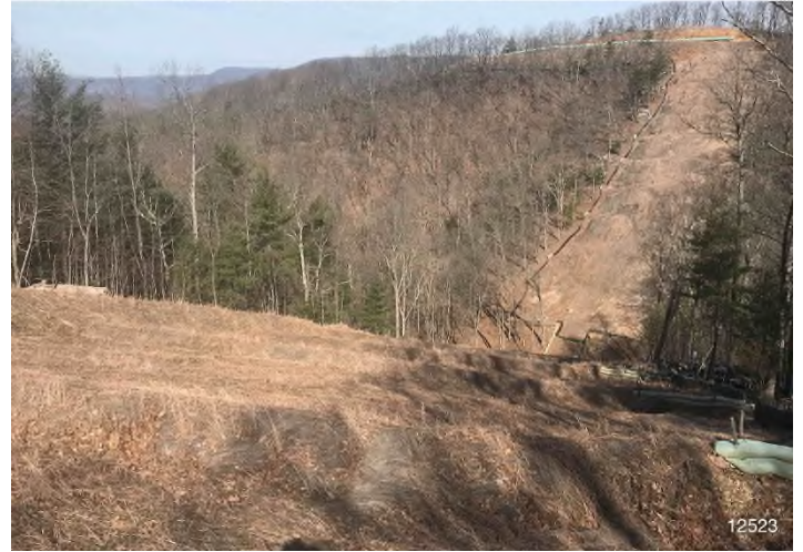
Figure 4: STA 12502+00 – Controls in place and functioning properly. Area stabilized with erosion control matting.
