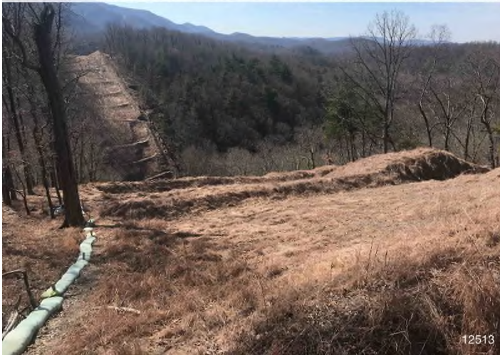
Figure 3: STA 12513+00 – Controls in place and functioning properly. Area stabilized with erosion control matting.
