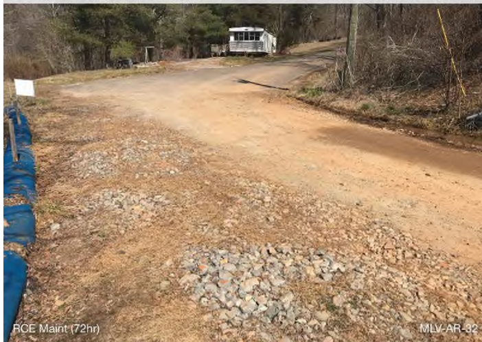
Figure 3: MLV-AR-32 – RCE maintenance needed.
