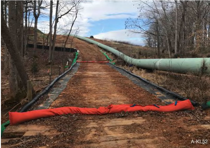
Figure 3: Stream S-KL54 – Controls in place and functioning properly. Area stabilized with straw and hydro-mulch.
