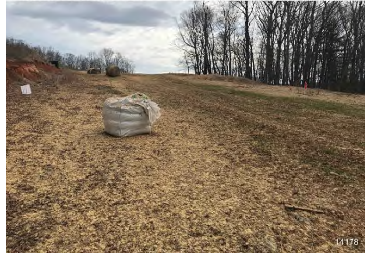
Figure 4: STA 14200+00 – Controls in place and functioning properly. Area stabilized with straw and hydro-mulch.
