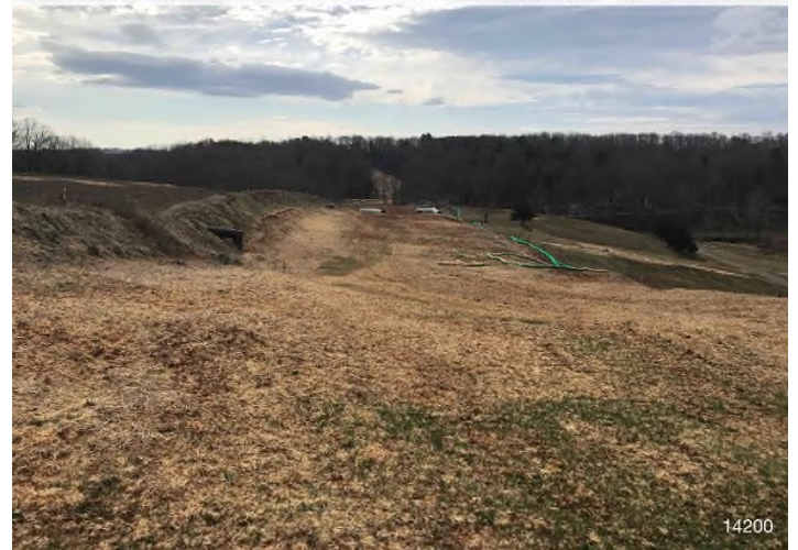
Figure 4: STA 14200+00 – Controls in place and functioning properly. Area stabilized with straw and hydro-mulch.
