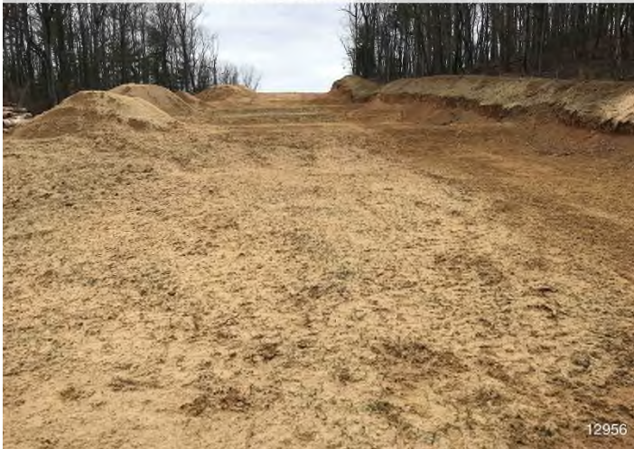
Figure 3: STA 12956+00 – Controls in place and functioning properly. Area stabilized with hydro-mulch and straw. BRG: 333°NW (T) LAT: 37.134928 LON: -80.137904 ±16ft ALT: 2648ft
