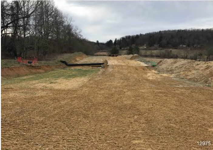
Figure 1: STA 12975+00 – Controls in place and functioning properly. Area stabilized with hydro-mulch and straw. BRG: 142°SE (T) LAT: 37.130313 LON: -80.136784 ±16ft ALT: 2680ft
