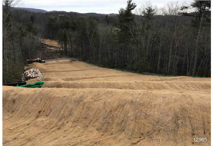
Figure 2: STA 12965+00 – Controls in place and functioning properly. Area stabilized with erosion control matting. BRG: 14°N (T) LAT: 37.132431 LON: -80.137334 ±98ft ALT: 2758ft
