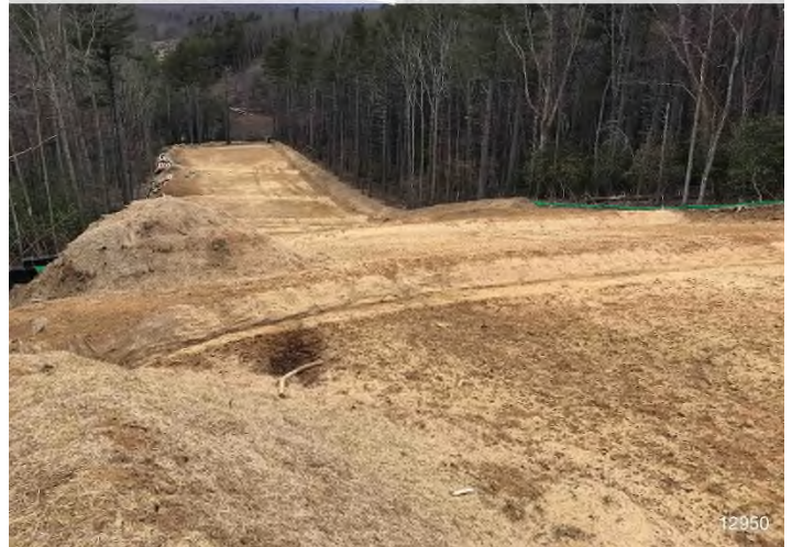
Figure 4: STA 12950+00 – Controls in place and functioning properly. Area stabilized with hydro-mulch and straw. BRG: 358°N (T) LAT: 37.146534 LON: -80.124510 ±7851ft ALT: 2640ft
