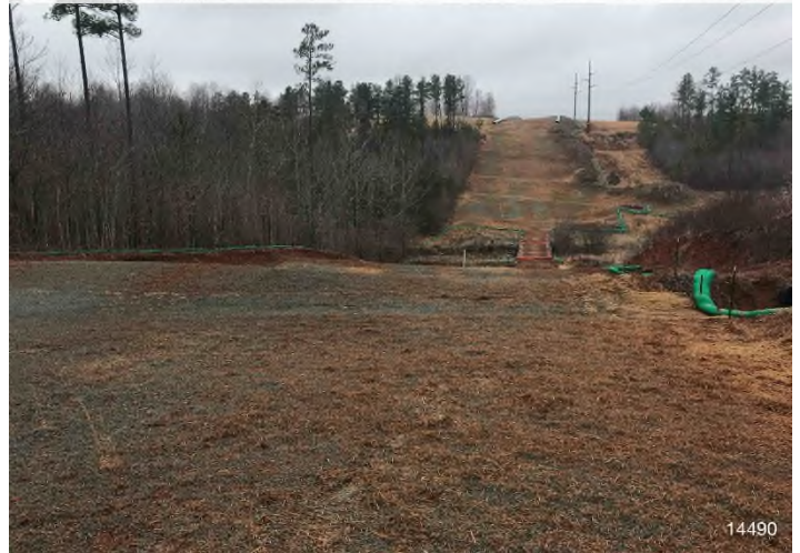
Figure 4: STA 14445+00 – Controls in place and functioning properly. Area stabilized with straw and Earth-Guard.
