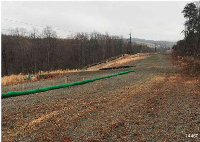
Figure 3: STA 14413+00 – Controls in place and functioning properly. Area stabilized with straw and Earth-Guard.
