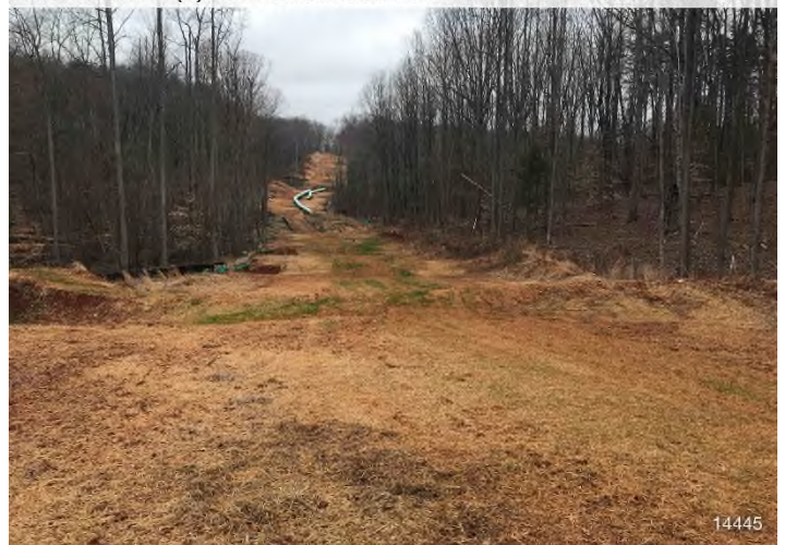
Figure 4: STA 14445+00 – Controls in place and functioning properly. Area stabilized with straw and Earth-Guard.
