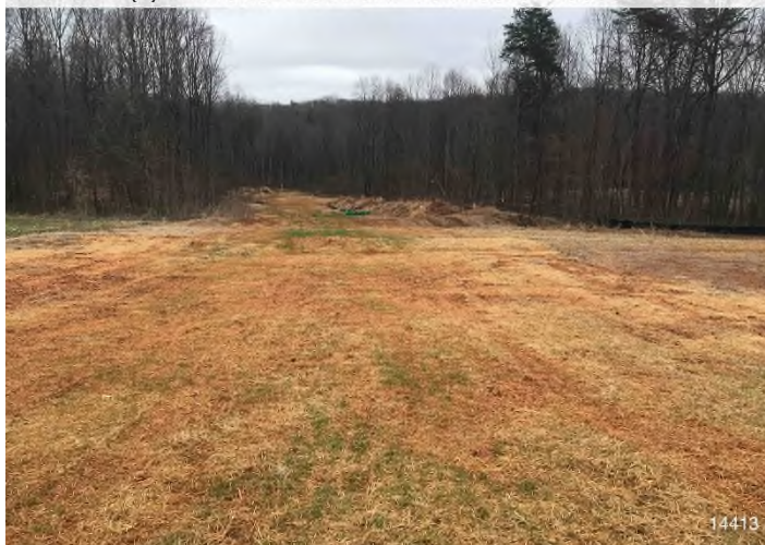
Figure 3: STA 14413+00 – Controls in place and functioning properly. Area stabilized with straw and Earth-Guard.
