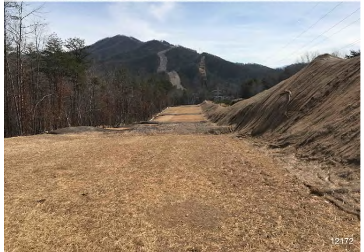
Figure 4: STA 12172+00 – Controls in place and functioning properly. Area stabilized with erosion control matting and straw. BRG: 99°E (T) LAT: 37.231655 LON: -80.260382 ±7205ft ALT: 1420ft
