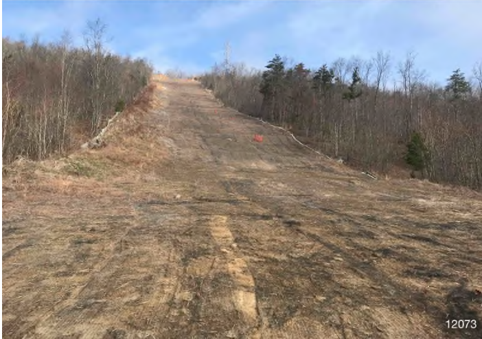
Figure 1: STA 12073+00 – Controls in place and functioning properly. Area stabilized with erosion control matting and straw. BRG: 357°N (T) LAT: 37.230819 LON: -80.260627 ±7205ft ALT: 1297ft
