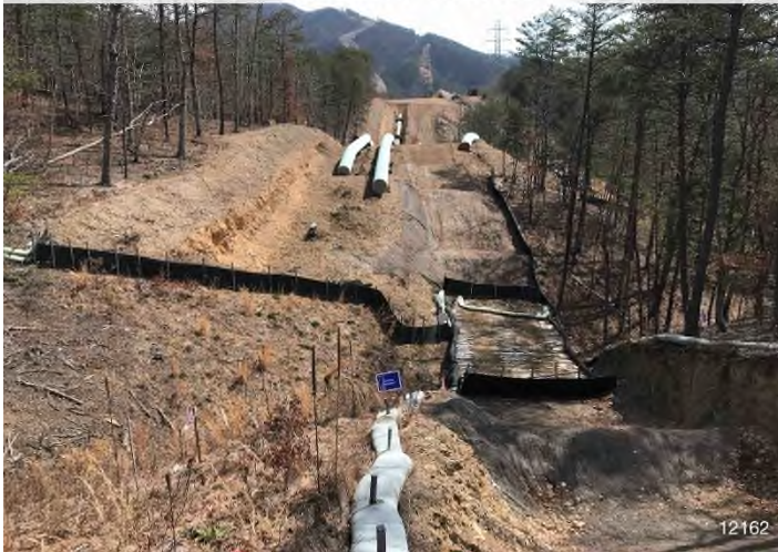
Figure 3: STA 12162+00 – Controls in place and functioning properly. Area stabilized with erosion control matting and straw. BRG: 98°E (T) LAT: 37.250842 LON: -80.267059 ±3051ft ALT: 1447ft
