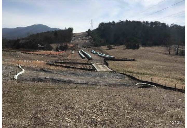
Figure 2: STA 12138+00 – Controls in place and functioning properly. Area stabilized with erosion control matting and straw. BRG: 102°E (T) LAT: 37.256126 LON: -80.276270 ±16ft ALT: 1420ft
