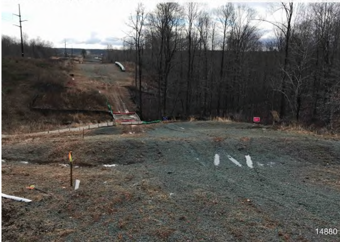
Figure 3: STA 14880+00 – Controls in place and functioning properly. Area stabilized with straw and Earth-Guard.
