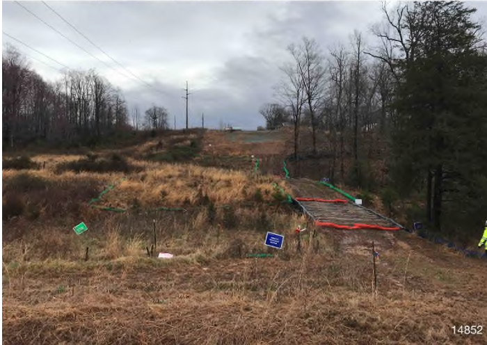
Figure 3: STA 14880+00 – Controls in place and functioning properly. Area stabilized with straw and Earth-Guard.
