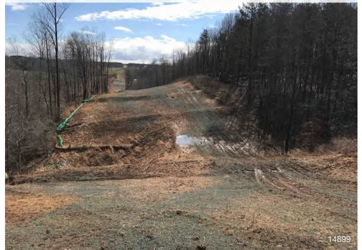
Figure 4: STA 14899+00 – Controls in place and functioning properly. Area stabilized with straw and Earth-Guard.
