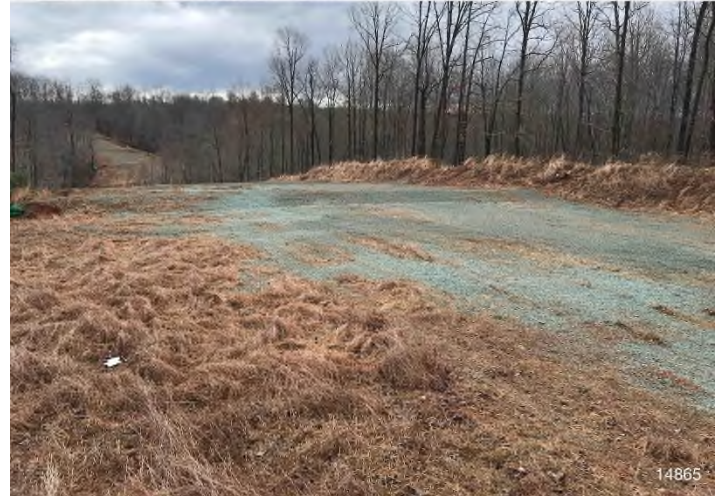
Figure 4: STA 14899+00 – Controls in place and functioning properly. Area stabilized with straw and Earth-Guard.
