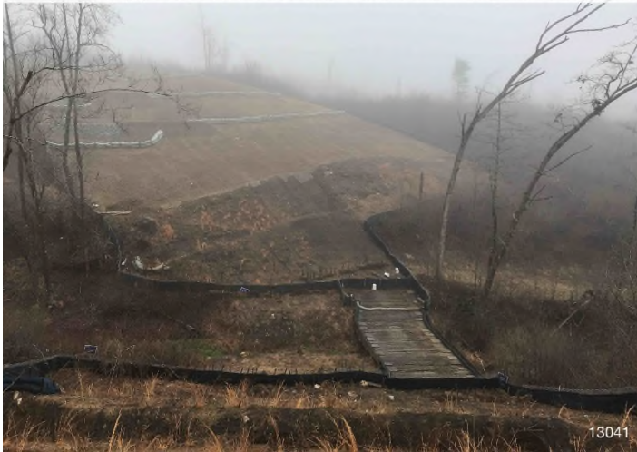
Figure 3: STA 13041+00 – Controls in place and functioning properly. BRG: 133°SE (T) LAT: 37.115051 LON: -80.077529 ±16421ft ALT: 2763ft
