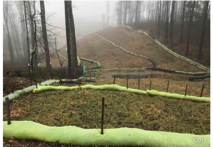
Figure 2: STA 13017+00 – Controls in place and functioning properly. BRG: 101°E (T) LAT: 37.125474 LON: -80.122712 ±164ft ALT: 3019ft
