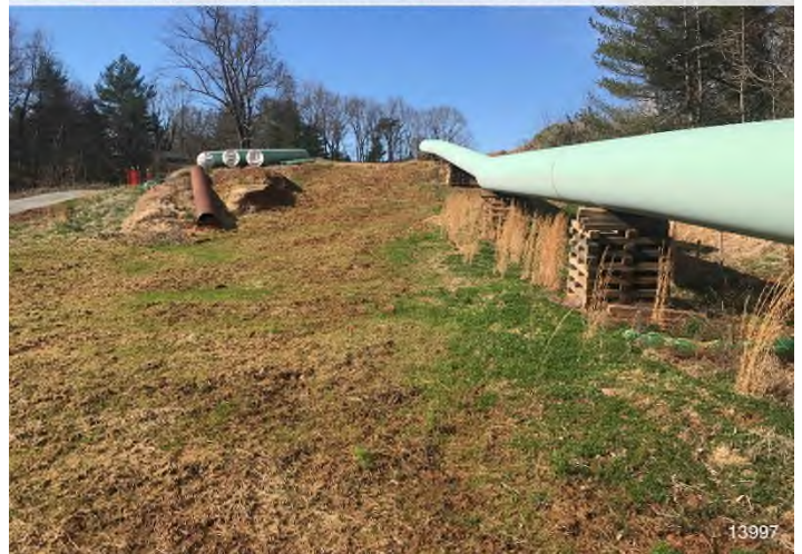
Figure 4: STA 13997+00 – Controls in place and functioning properly. Area stabilized with straw and Earth-Guard Edge.
