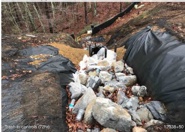
Figure 3: STA 12338+50 – Trash and construction debris deposited in controls.
