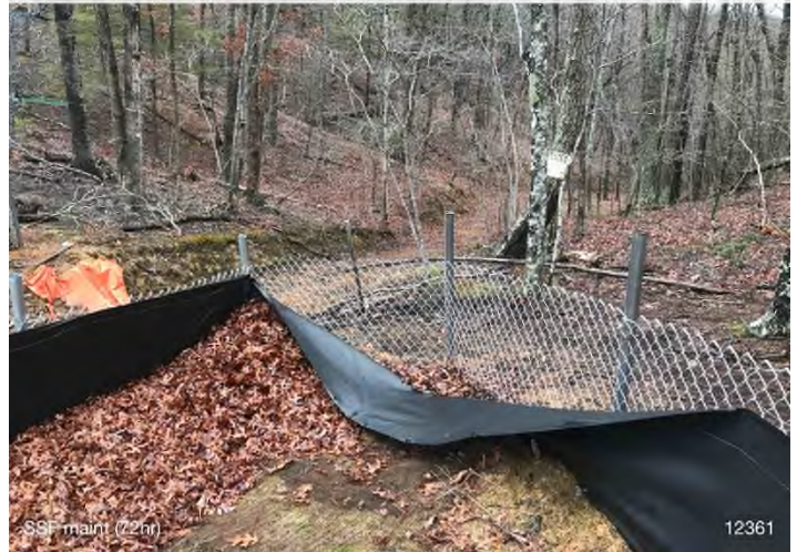
Figure 4: STA 12352+00 – Construction debris deposited off ROW.
