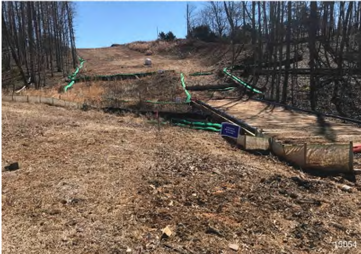
Figure 7: STA 15054+00 – Controls in place and functioning properly. Area stabilized with straw and erosion matting. No erosion evident.
