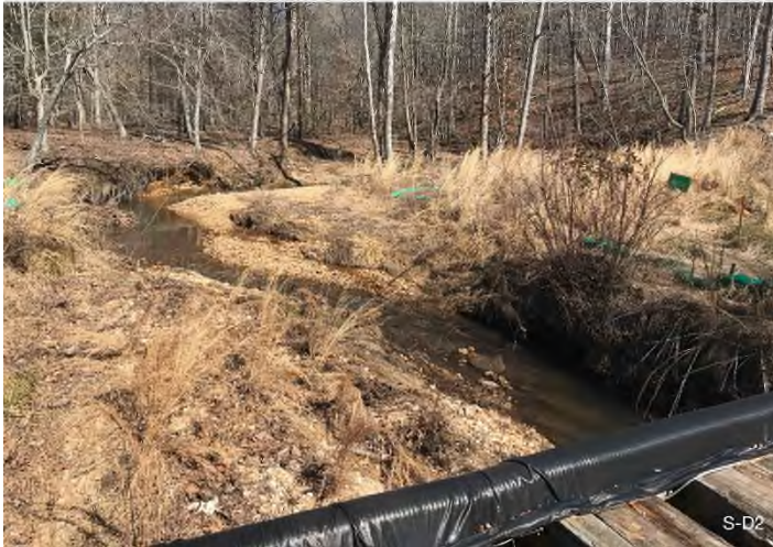
Figure 7: STA 15054+00 – Controls in place and functioning properly. Area stabilized with straw and erosion matting. No erosion evident.
