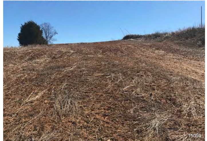
Figure 8: STA 15059+00 – Controls in place and functioning properly. Area stabilized with straw and erosion matting. No erosion evident.
