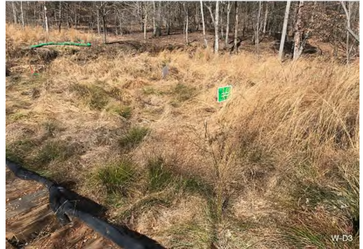
Figure 8: STA 15059+00 – Controls in place and functioning properly. Area stabilized with straw and erosion matting. No erosion evident.
