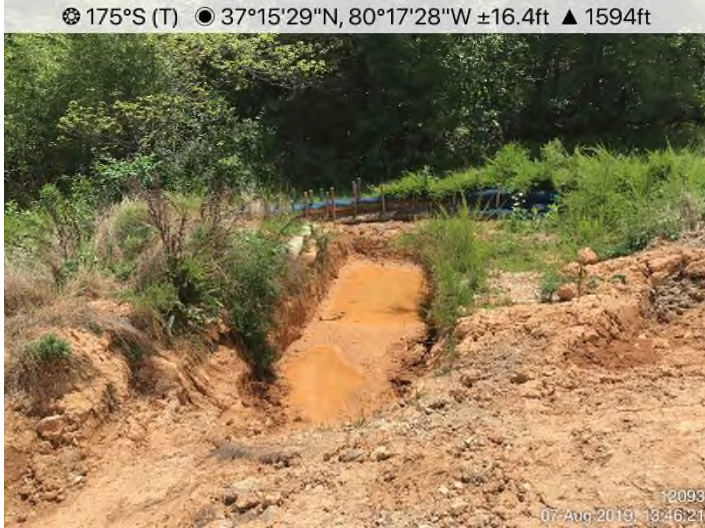
Fig. 3: STA 12093+00 – Sump maintenance needed.
