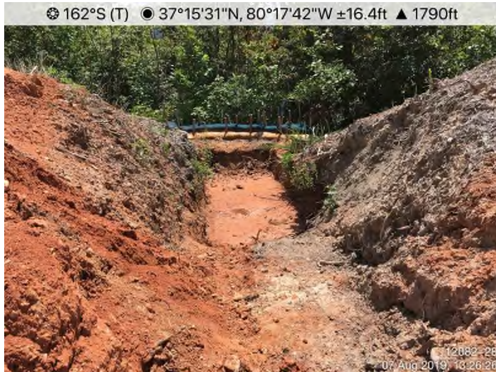
Fig. 3: STA 12093+00 – Sump maintenance needed.
