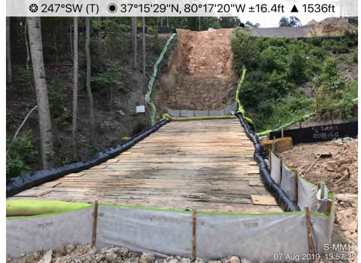
Fig. 4: Stream S-MM13 – Perimeter controls in place. Bridge clean and sideboards in place and functioning.
