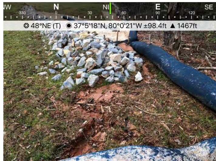
Fig. 3: STA 13497 – CFS undermined. CFS full.
