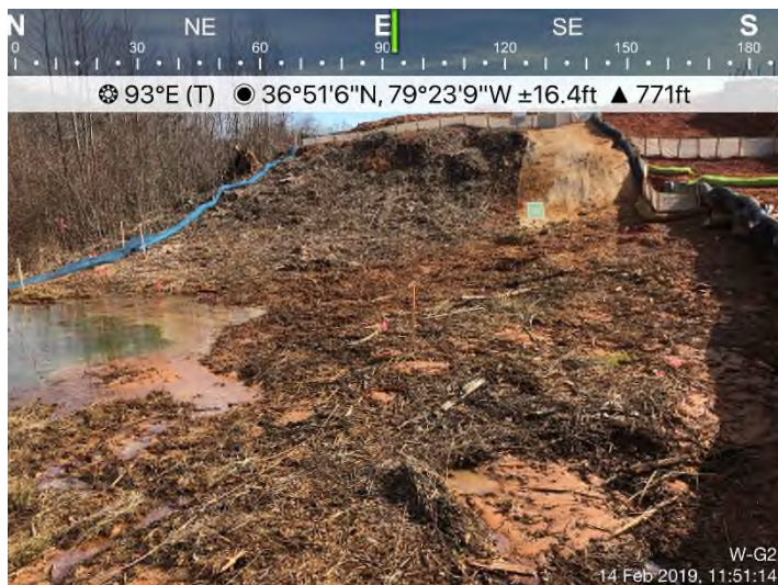
Fig. 7: W-G2 – Sediment deposition in wetland at STA 15852+59
