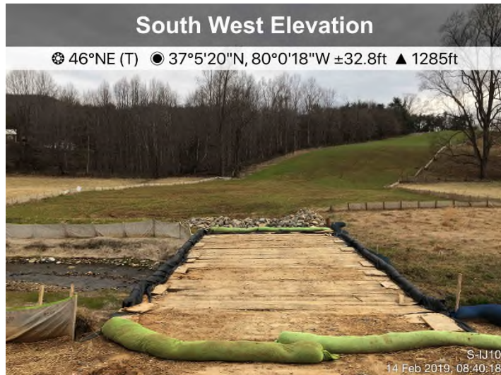
Fig. 3: STA 13497 – CFS undermined. CFS full.
