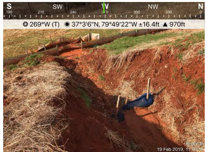
Fig. 4: STA 14273+25 – Clean out CFS.
