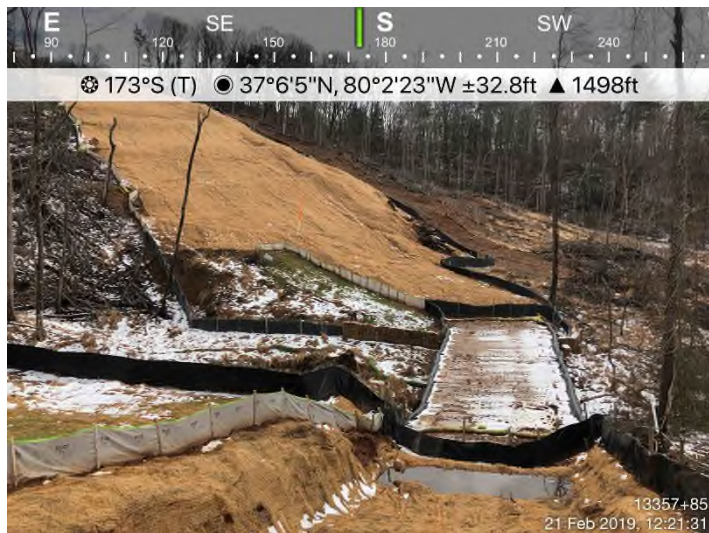
Fig. 7: STA 13357+85 – S-R11 controls in place. Area stabilized.
