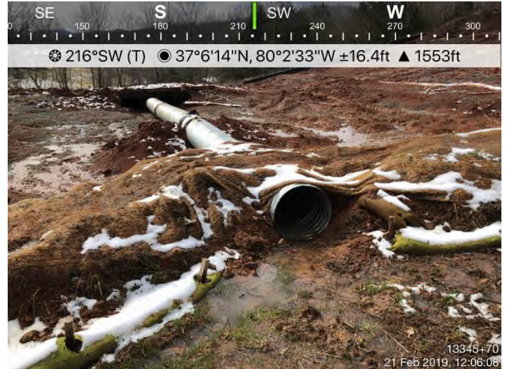
Fig. 4: STA 13345+70 – Inlet protection needed.
