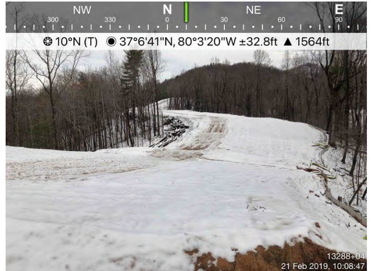
Fig. 4: STA 13345+70 – Inlet protection needed.
