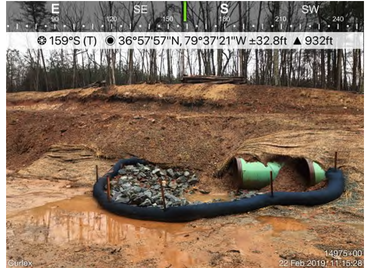
Fig. 4: STA 14975+00 – Erosion fabric maintenance.
