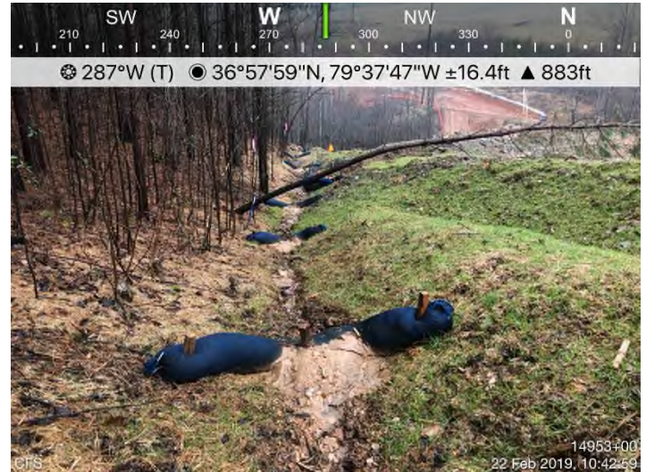
Fig. 4: STA 14975+00 – Erosion fabric maintenance.
