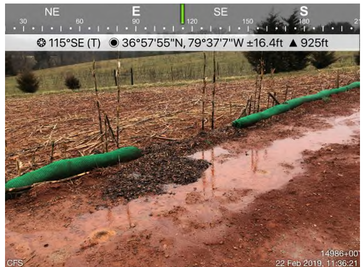
Fig. 8: STA 14986+00 – CFS maintenance needed.
