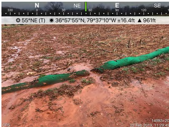
Fig. 7: STA 14983+20 – CFS maintenance needed.
