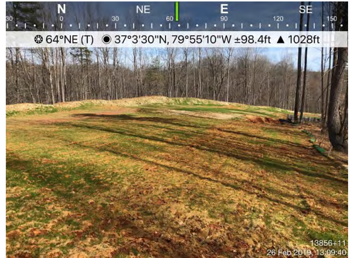
Fig. 10: STA 13856+11 – Area stabilized. Controls in place.
