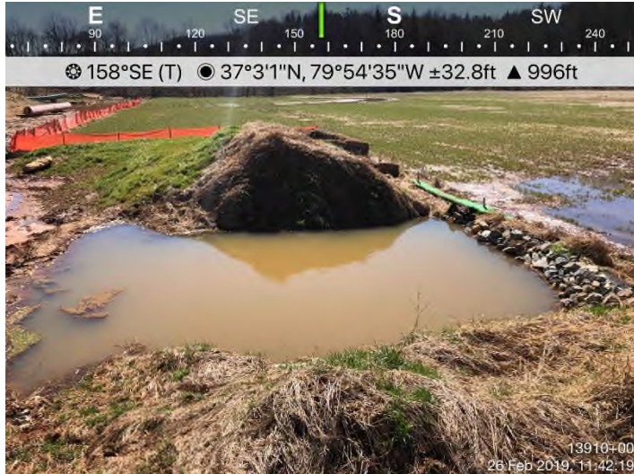
Fig. 3: STA 13910+00 – CWD unable to drain.
