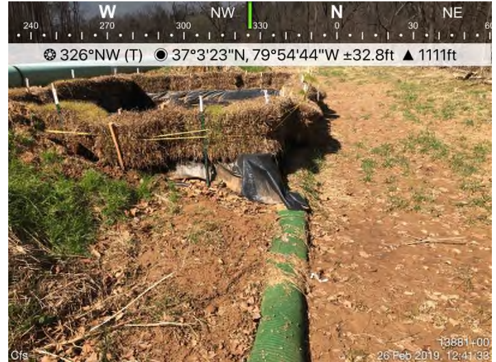
Fig. 8: STA 13881+00 – CFS needs maintenance.
