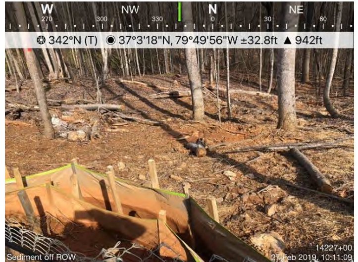
Fig. 12: STA 14231+50 – Sumps need maintenance.
