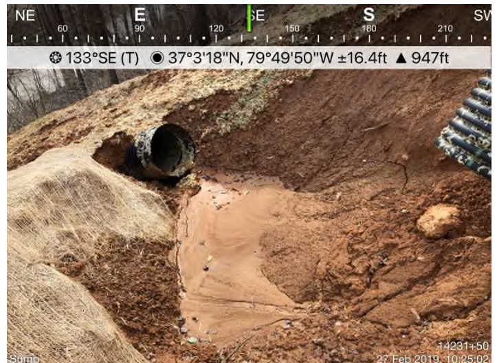
Fig. 12: STA 14231+50 – Sumps need maintenance.
