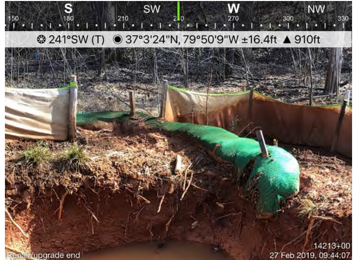
Fig. 4: STA 14213+00 – Maintain CFS/upgrade end-treatment.
