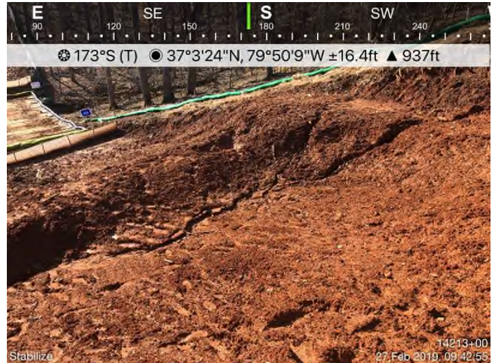
Fig. 4: STA 14213+00 – Maintain CFS/upgrade end-treatment.
