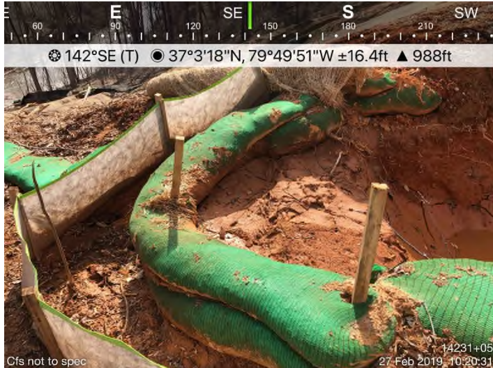
Fig. 11: STA 14331+05 – P1 undermined, CFS not installed per spec., sump full.
