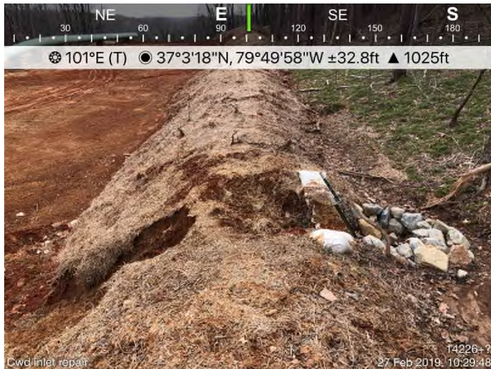
Fig. 11: STA 14331+05 – P1 undermined, CFS not installed per spec., sump full.
