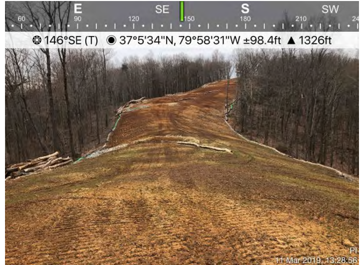
Fig. 8: STA 13590 – ROW at final grade.
