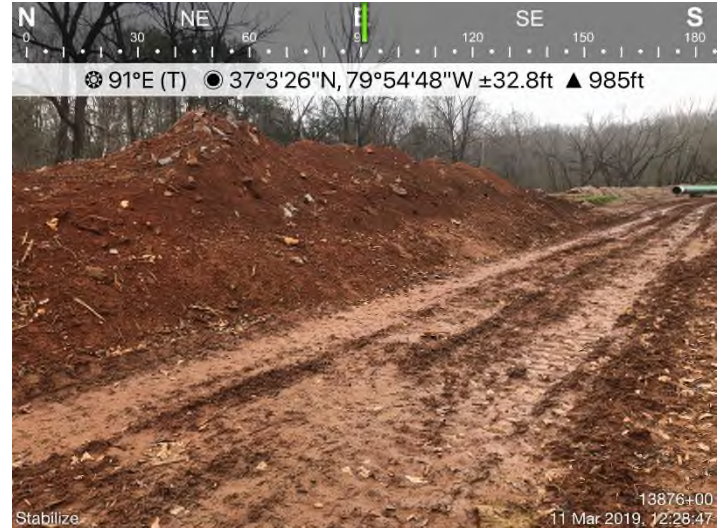
Fig. 4: STA 13876+00 – Stabilization needed on stockpiles.
