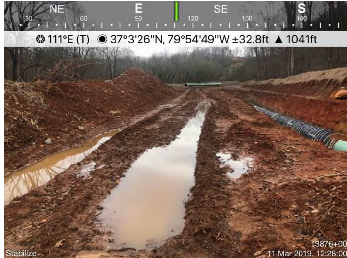
Fig. 3: STA 13879+00 – ROW stabilization needed.
