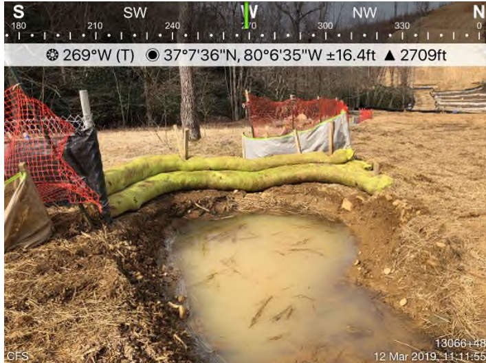
Fig. 7: STA 13066+48 – CFS undermined. Maintenance needed.
