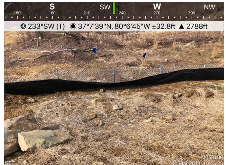
Fig. 4: STA 13058+00 – Maintenance needed on SSF.
