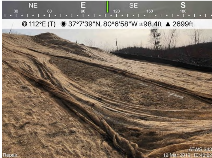
Fig. 3: ATWS 343 – Maintenance needed on fabric.
