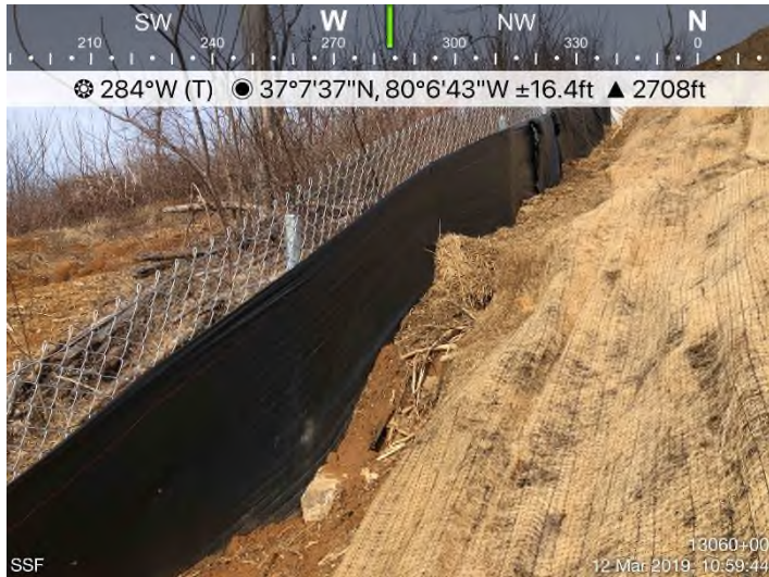
Fig. 7: STA 13066+48 – CFS undermined. Maintenance needed.
