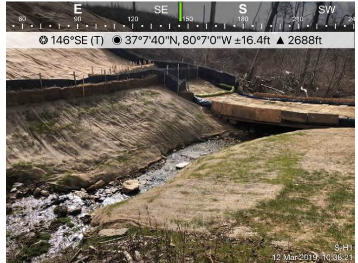
Fig. 4: STA 13058+00 – Maintenance needed on SSF.
