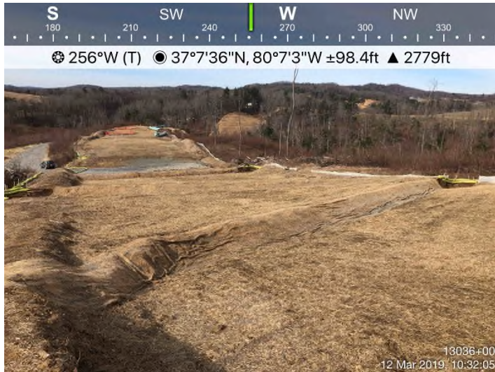
Fig. 3: ATWS 343 – Maintenance needed on fabric.
