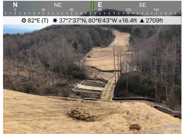
Fig. 8: MVP-FR-290 – Area adequately stabilized. Controls in place.
