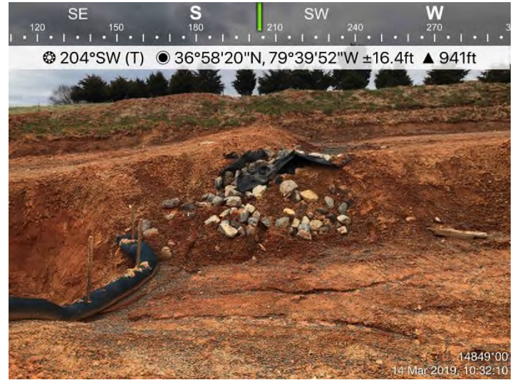
Fig. 4: STA 14852+00 – Repair/maintain end treatment.
