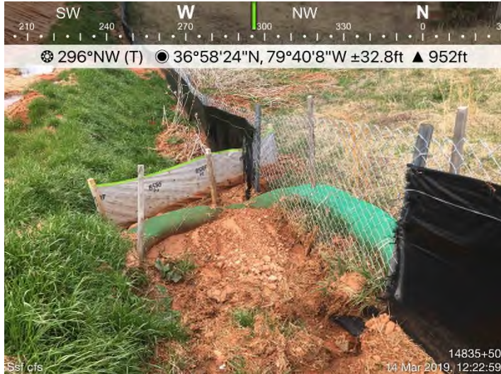
Fig. 15: STA 14835+50 – Clean out/maintain CFS. Repair SSF.
