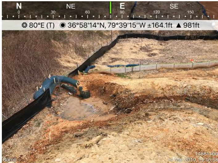
Fig. 15: STA 14835+50 – Clean out/maintain CFS. Repair SSF.
