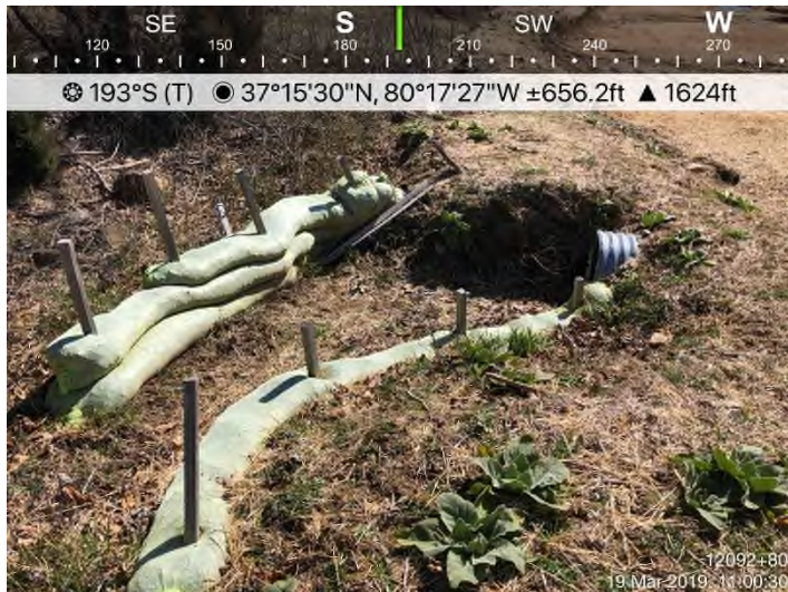
Fig. 7: STA 12100+00 – Perimeter CWD berm failing.
