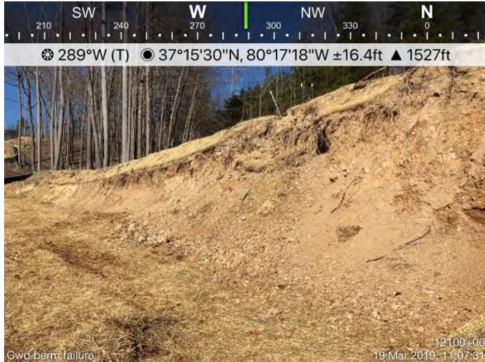
Fig. 7: STA 12100+00 – Perimeter CWD berm failing.
