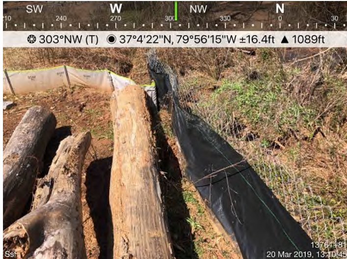
Fig. 3: STA 13761+87 – SSF undermined.
