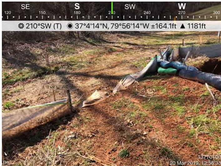
Fig. 3: STA 13761+87 – SSF undermined.
