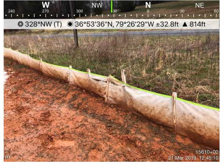
Fig. 8: STA 15611+66 - Repair CFS.
