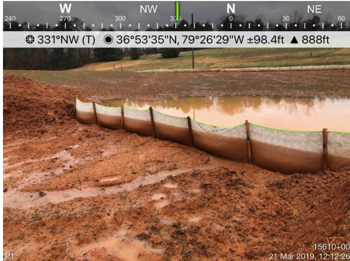
Fig. 7: STA 15610+00 - P1 Undermined, clean out CFS.
