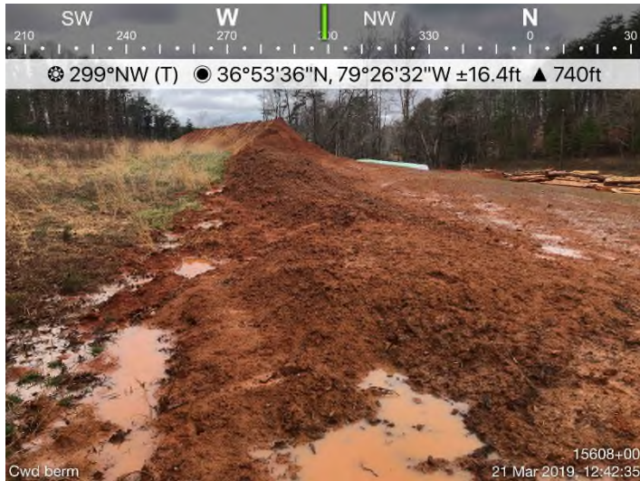
Fig. 7: STA 15610+00 - P1 Undermined, clean out CFS.
