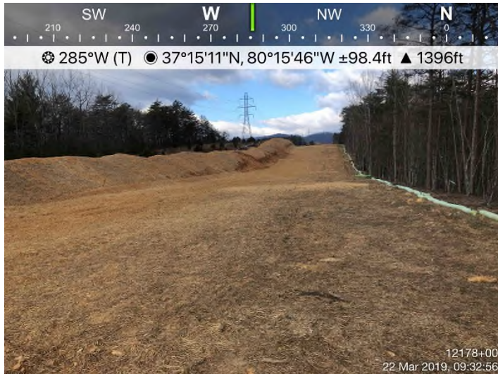
Fig. 3: STA 12161+00 – Area adequately stabilized. Controls in place.
