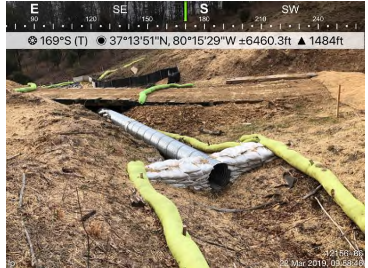
Fig. 4: STA 12156+86 – CWD needs inlet protection.
