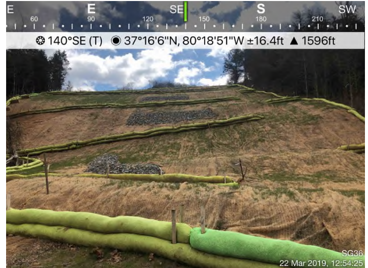
Fig. 8: STA 12008+53 – Area adequately stabilized. Controls in place.
