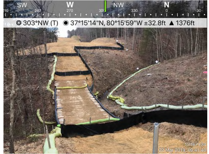
Fig. 4: STA 12156+86 – CWD needs inlet protection.
