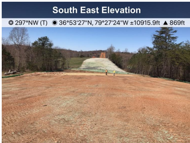
Fig. 11 Near MP287 final restoration in process
