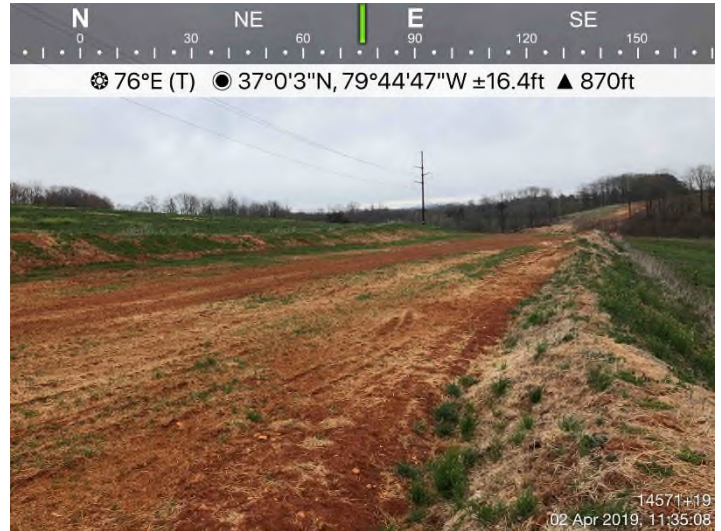
Fig. 4: STA 14549+84 – CWD does not have inlet protection.
