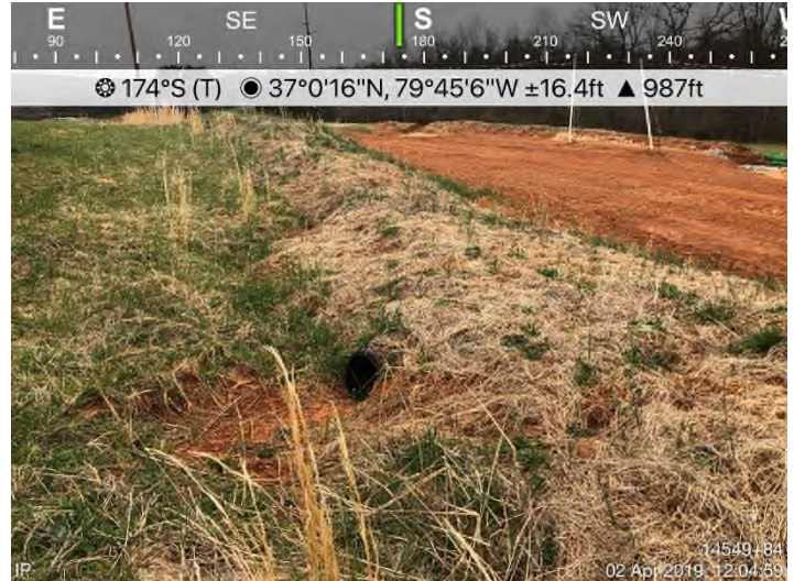
Fig. 4: STA 14549+84 – CWD does not have inlet protection.
