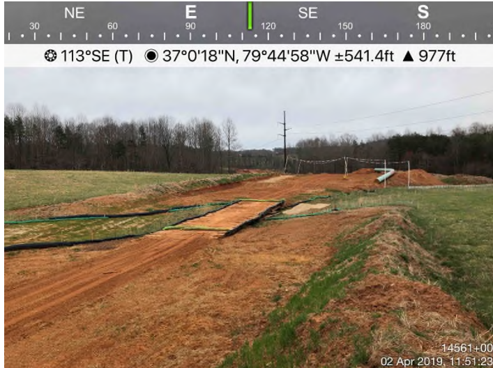
Fig. 3: STA 14561+00 – Area adequately stabilized. Controls in place.
