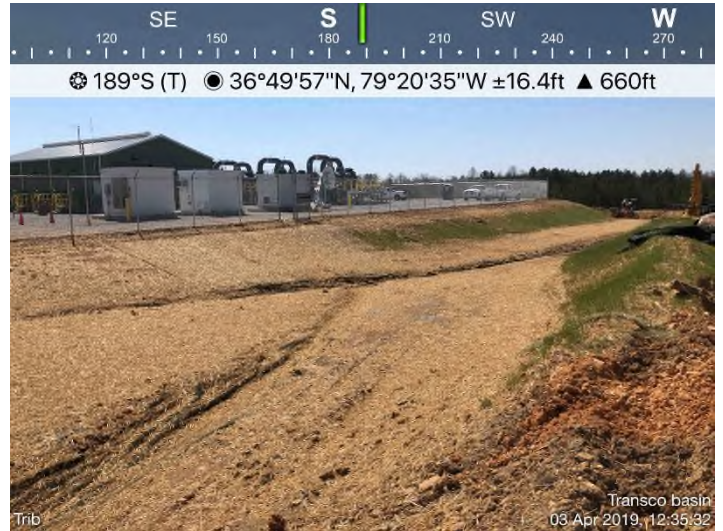
Fig. 4: Permanent Stormwater Pond – Inlet channel K (CH-K).
