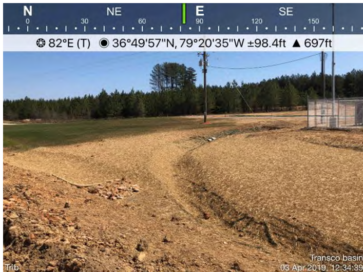
Fig. 3: Permanent Stormwater Pond – Inlet channel J (CH-J).
