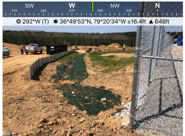
Fig. 4: Permanent Stormwater Pond – Inlet channel K (CH-K).
