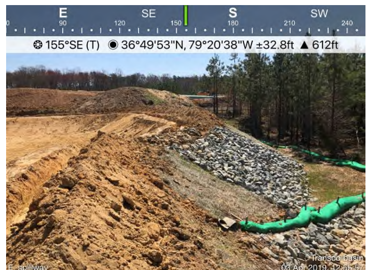
Fig. 8: Permanent Stormwater Pond – Emergency spillway.
