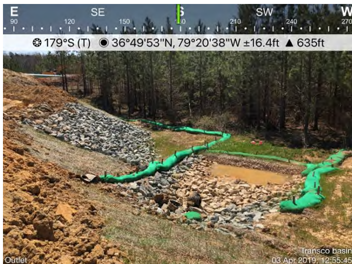
Fig. 7: Permanent Stormwater Pond – Outfall.
