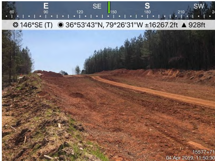
Fig. 3: STA 15555+00 – Area adequately stabilized with Earth Guard. Controls in place.
