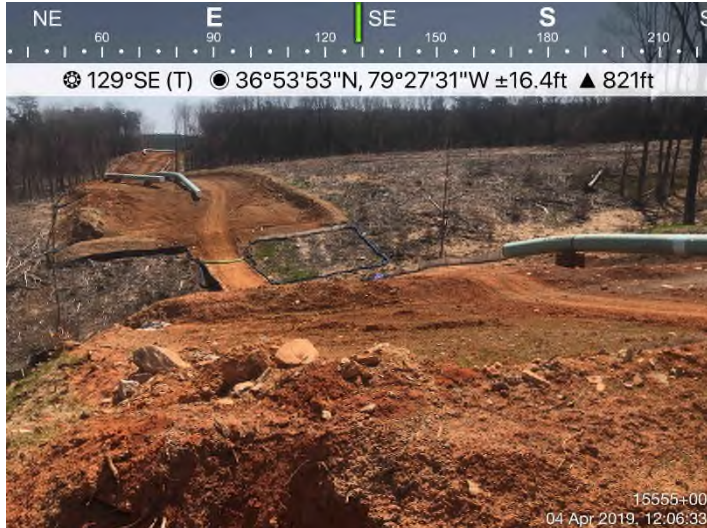
Fig. 3: STA 15555+00 – Area adequately stabilized with Earth Guard. Controls in place.
