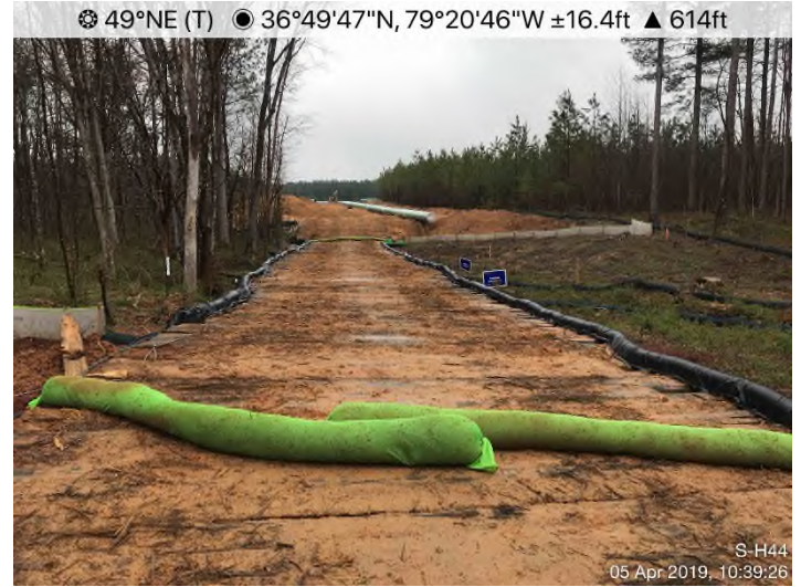
Fig. 8: H-602 STA 11+96 – Area adequately stabilized with Earth Guard. Controls in place.
