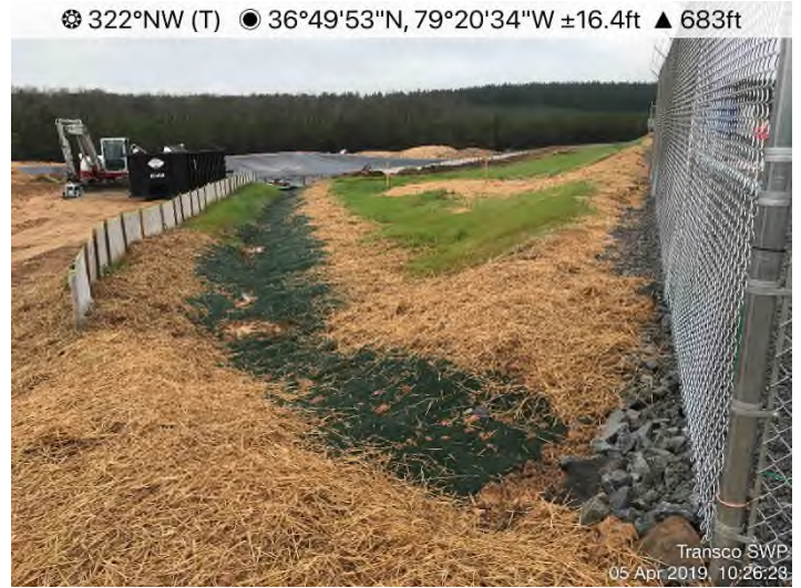
Fig. 4: Transco Stormwater Pond – Liner and baffle installation.
