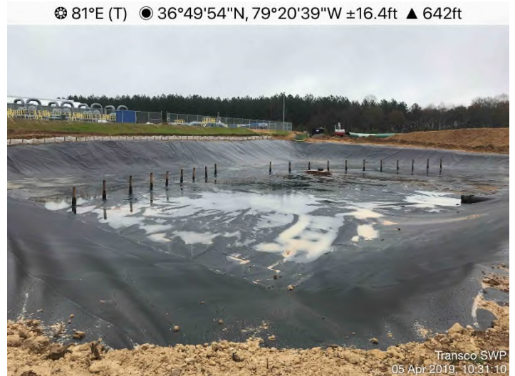
Fig. 4: Transco Stormwater Pond – Liner and baffle installation.
