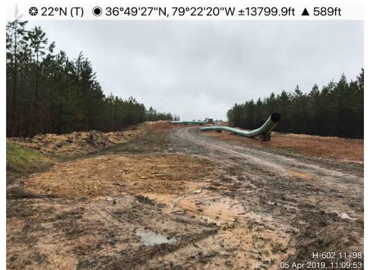
Fig. 8: H-602 STA 11+96 – Area adequately stabilized with Earth Guard. Controls in place.
